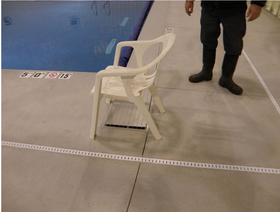
Trip hazards throughout the pool decking
