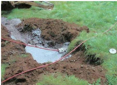
Removing Contaminated Sludge
