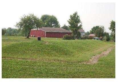
Simply, a mound is a bed elevated above one to two feet of clean sand. The sand will be extended to each side of the bed in order to create enough contact between the original soil and the system. Loamy soil and topsoil (1.5-2 feet) will be used as a cover.
